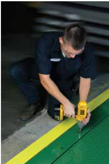
Engineer during installation at site
